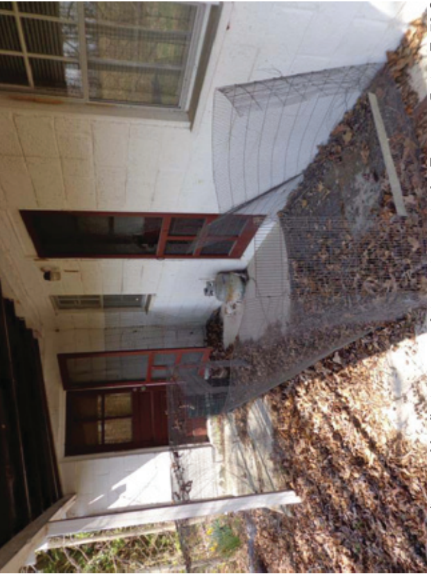
PHOTO 57: Empty Propane Tank at vacant care taker property (looking east)
