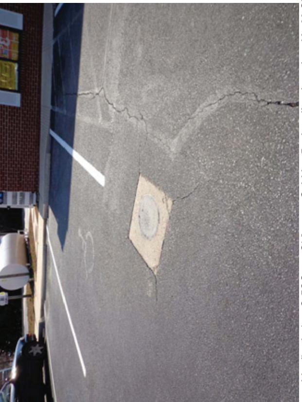
PHOTO 58: Abandoned well at the Dunkirk Sinoco (Open OCB Case) site (looking east)
