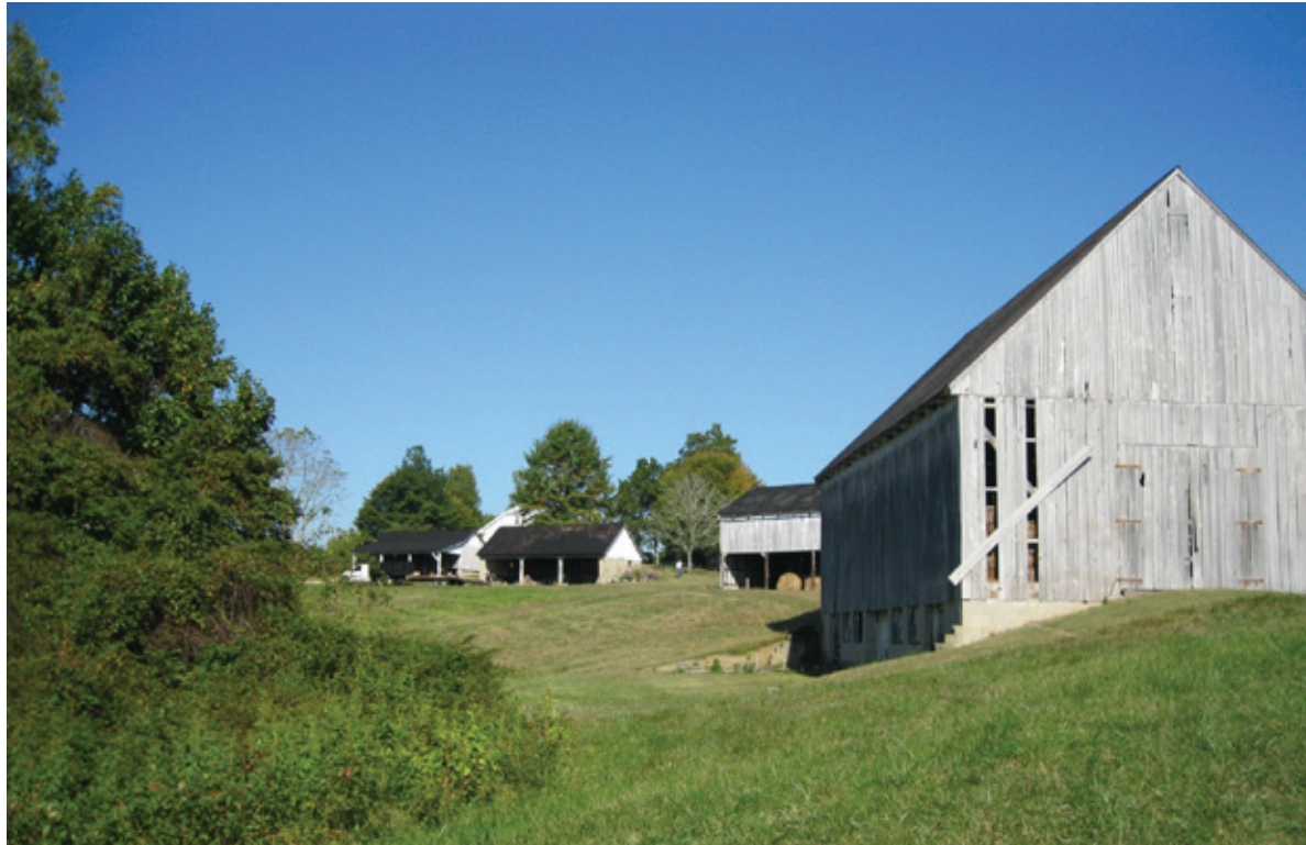
Existing structures on the site
