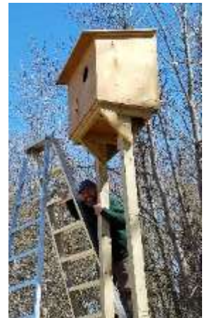
Newly installed box at Al Tucker's Farm March 2021
